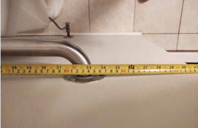
Photo AMN10 – Dwelling Unit C6 - Measured dimension to far edge of rear grab bar at 33” from the side wall.
