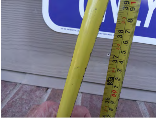
Photo CS1 – Measured height of 37 ½” to bottom of accessible sign.
