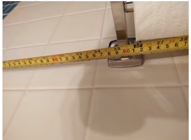
Photo CS4 – Unisex Toilet Room – Measured dimension of 35” to nearest edge of toilet paper dispenser to back wall.
