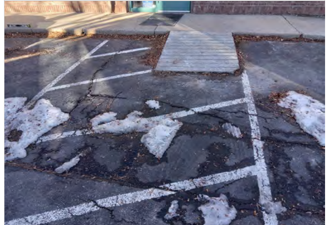
Photo CS2 – Curb ramp extending into the access aisle between accessible parking spaces.
