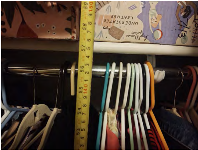
Photo L13 – Dwelling Unit #104 – Measured height to top of clothes rod at 56”.
