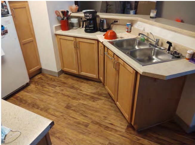
Photo L17 – Dwelling Unit #104 - Kitchen sink with permanent base cabinet.
