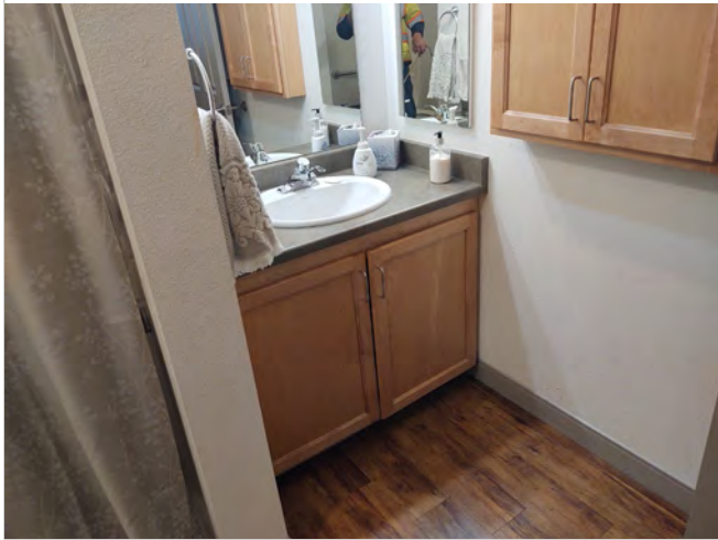
Photo L21 – Dwelling Unit #106 - Bathroom sink with permanent base cabinet.
