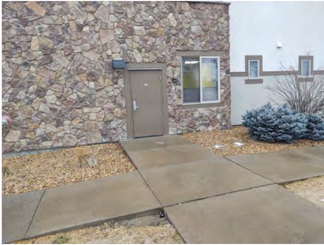
Photo L5 – Non-accessible side entrance door.
