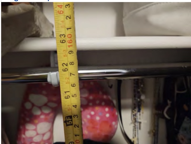
Photo L19 – Dwelling Unit #106 - Measured height to top of clothes rod at 62”.
