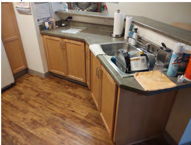
Photo L23 – Dwelling Unit #106 - Kitchen sink with permanent base cabinet
