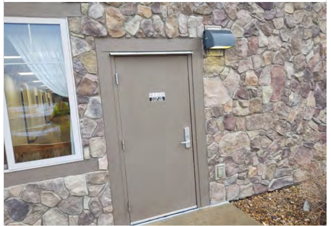
Photo L6 – Non-accessible side entrance door.
