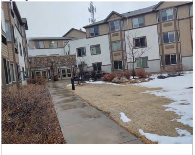
Photo L4 – Rear accessible entrance without signage.
