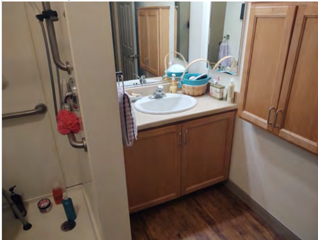
Photo L15 – Dwelling Unit #104 – Bathroom sink with permanent base cabinet.
