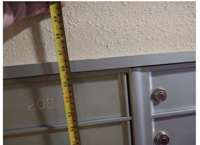
Photo L8 – Measured height to top of mailbox bank at 65 1/2”.
