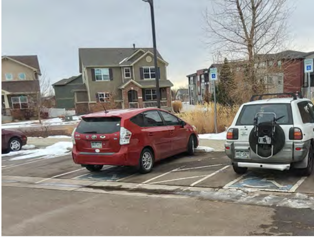
Photo SC1 – Access aisle at accessible parking spaces at south wing.
