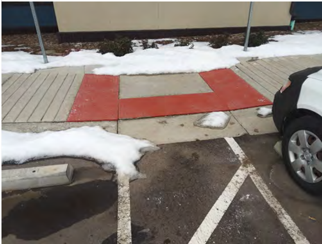
Photo SC3 – Access aisle at accessible parking spaces at south wing.
