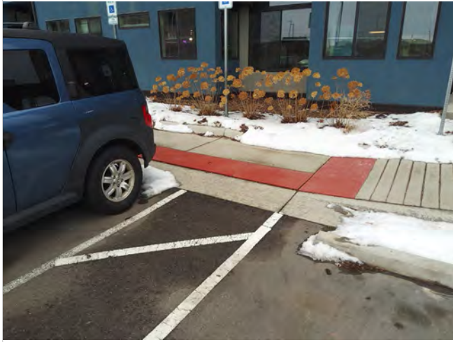
Photo SC5 – Access aisle at accessible parking spaces at east wing.
