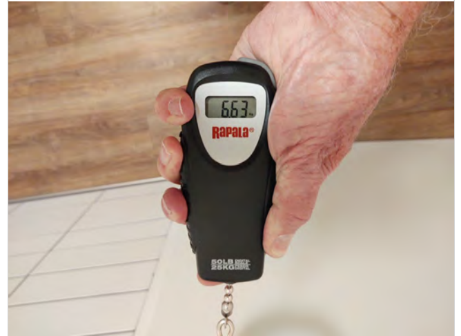
Photo FR12 – Fourth Level Unisex Toilet Room - Measured door pull of 6.63 lbs.
