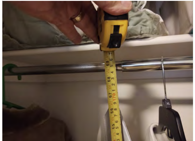
Photo FR18 – Dwelling Unit #207 - Measured height of 69” at clothes rod.
