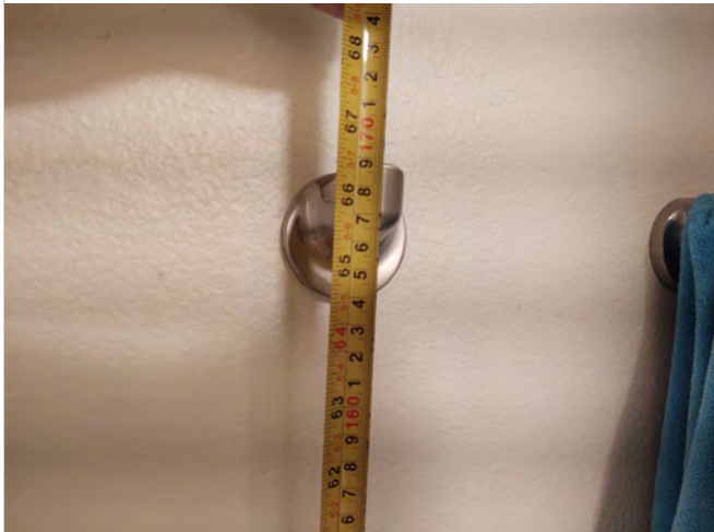
Photo FR21 – Dwelling Unit #207 - Measured height of 66" at coat hook.
