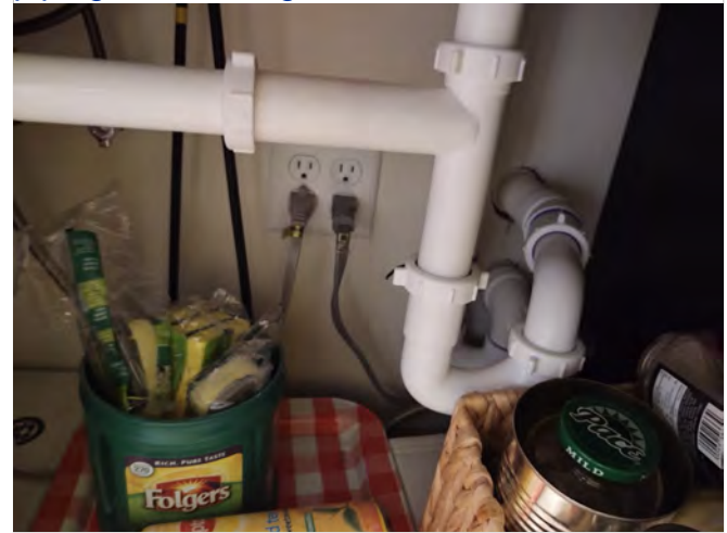
Photo FR24 – Dwelling Unit #212 - Exposed piping and flooring beneath Kitchen sink.
