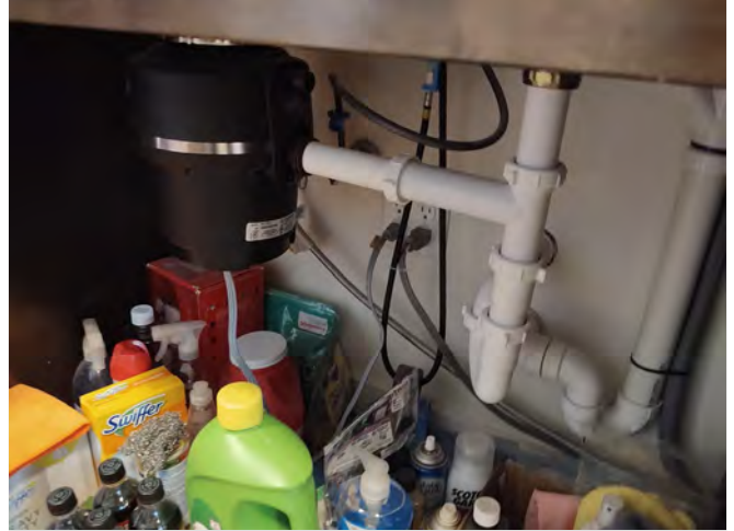
Photo FR26 – Dwelling Unit #414 - Exposed piping and flooring beneath Kitchen sink.
