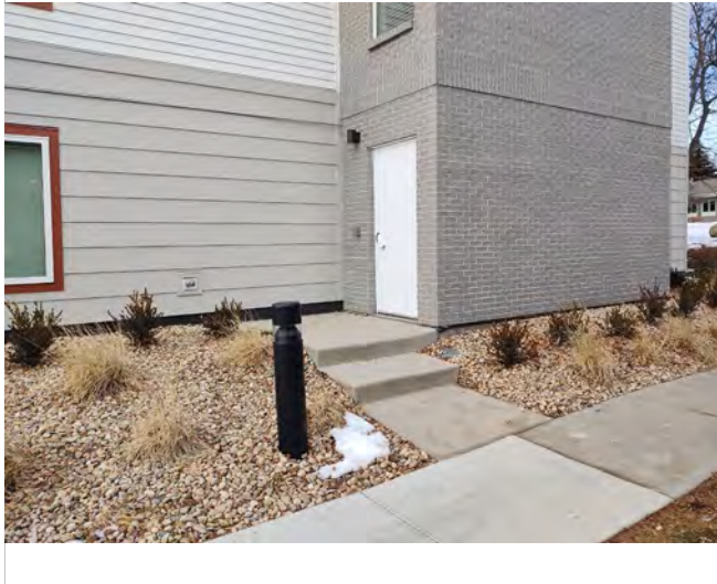
Photo AM3 – Non-accessible side door.
