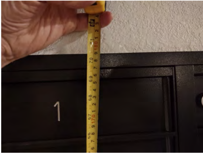
Photo AM5 – Measured height of 69 ½” to top of mailbox bank.
