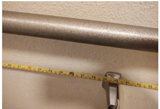
Photo B16 – Dwelling Unit #104 - Measured near edge of the toilet paper dispenser at 39” from the back wall.
