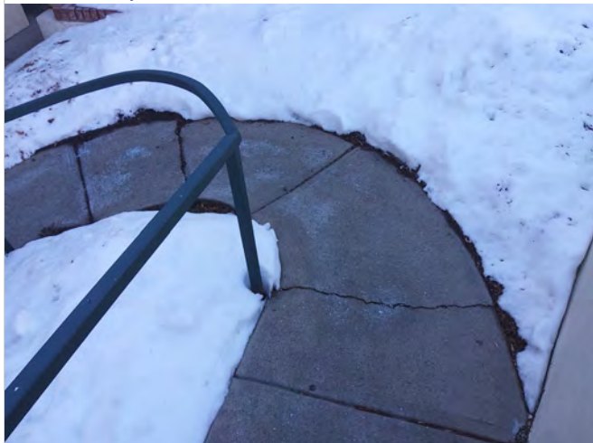
Photo B7 – Curve at middle of accessible route ramp.
