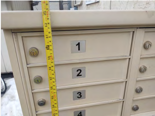
Photo B11 – Measure height to top of exterior bank of mailboxes is 61.”
