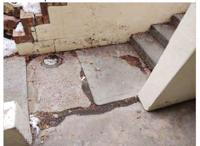
Photo B8 – Landing at bottom of accessible route ramp.
