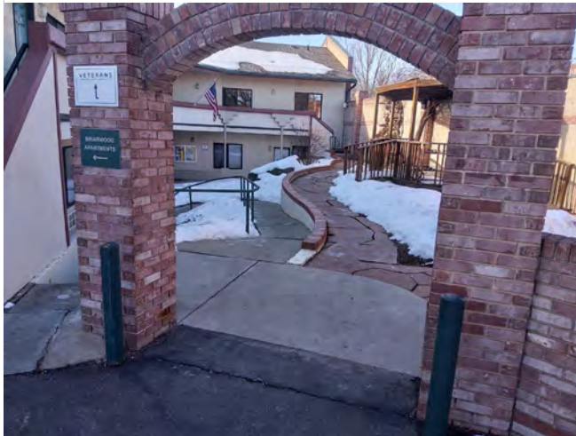
Photo B3 – Ramp at Accessible Route to lower level of dwelling units.
