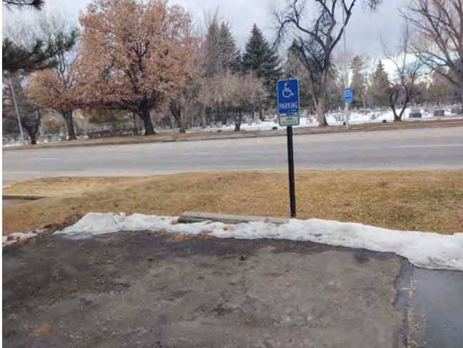
Photo CL1 – Signage in front of accessible parking space.
