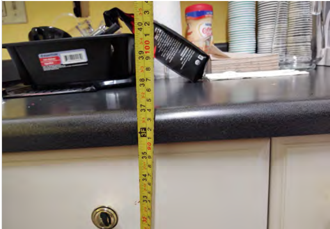
Photo CL9 – Kitchenette – Measured height of 37” to top of kitchen sink.
