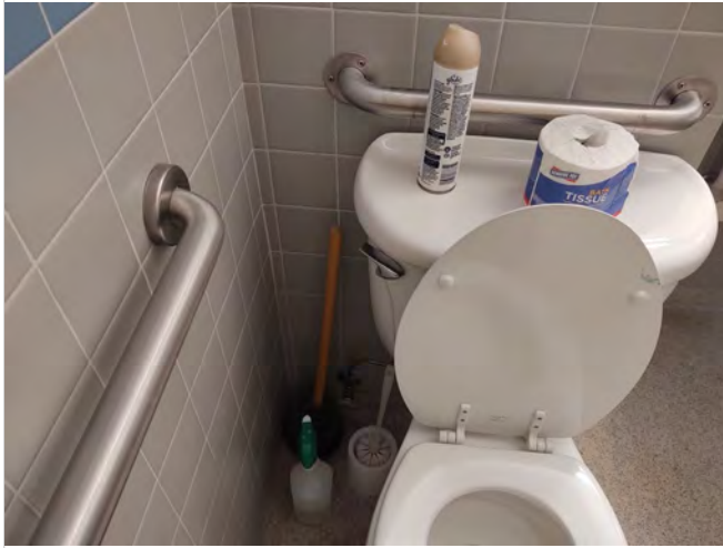
Photo CL5 – Unisex Toilet Room – Flush control on wall side of water closet.
